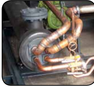
Yüksek Verimli Shell and Tube Evaporatör High Efficiency Shell and Tube Evaporator
